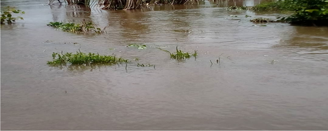
The road at Dzakpo after heavy rainfalls, making it impossible to reach the community (15/05/2021)
